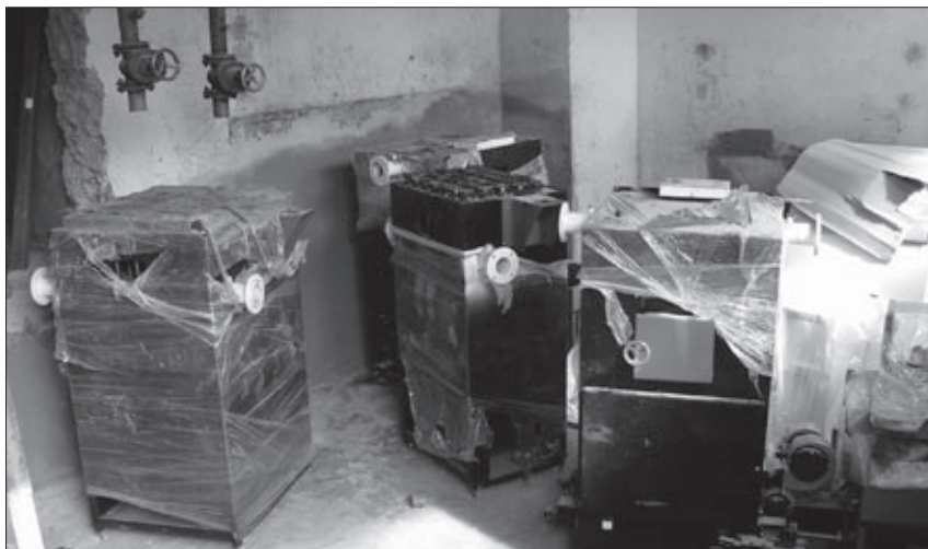
Boilers in Zákamenné ready to be installed
