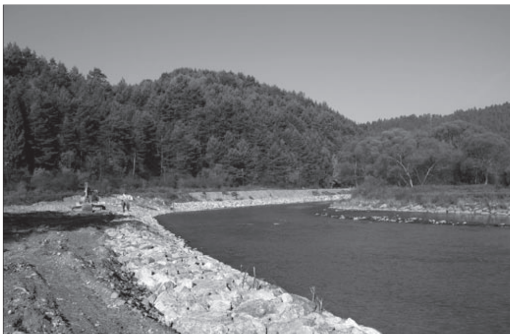
Stabilizing Poprad river banks in Stariná
